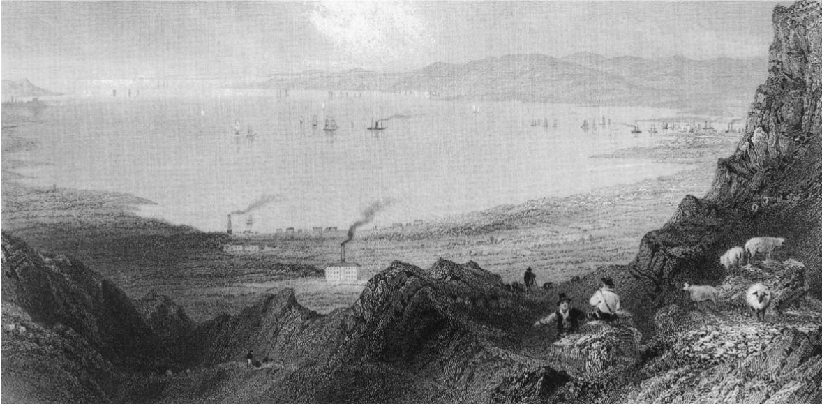
Nineteenth-century view of Belfast Lough.
