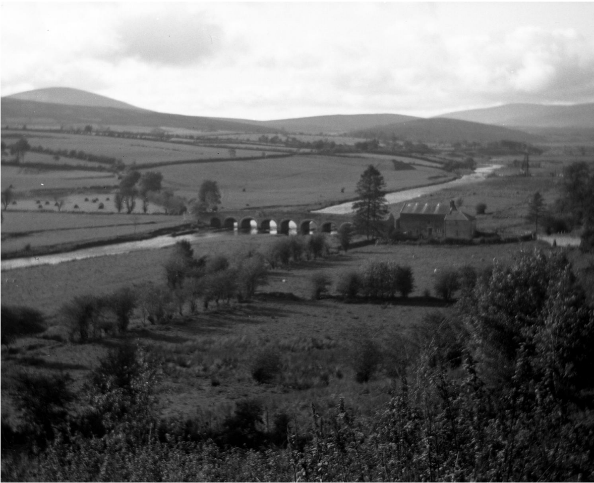
Blessington Bridge and the River Liffey, 1938.
