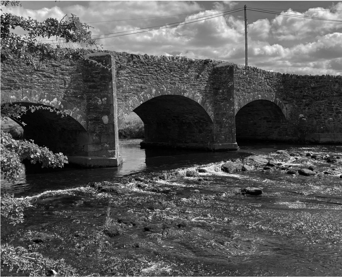
Ballyhubbock Bridge over the Slaney in County Wicklow.
